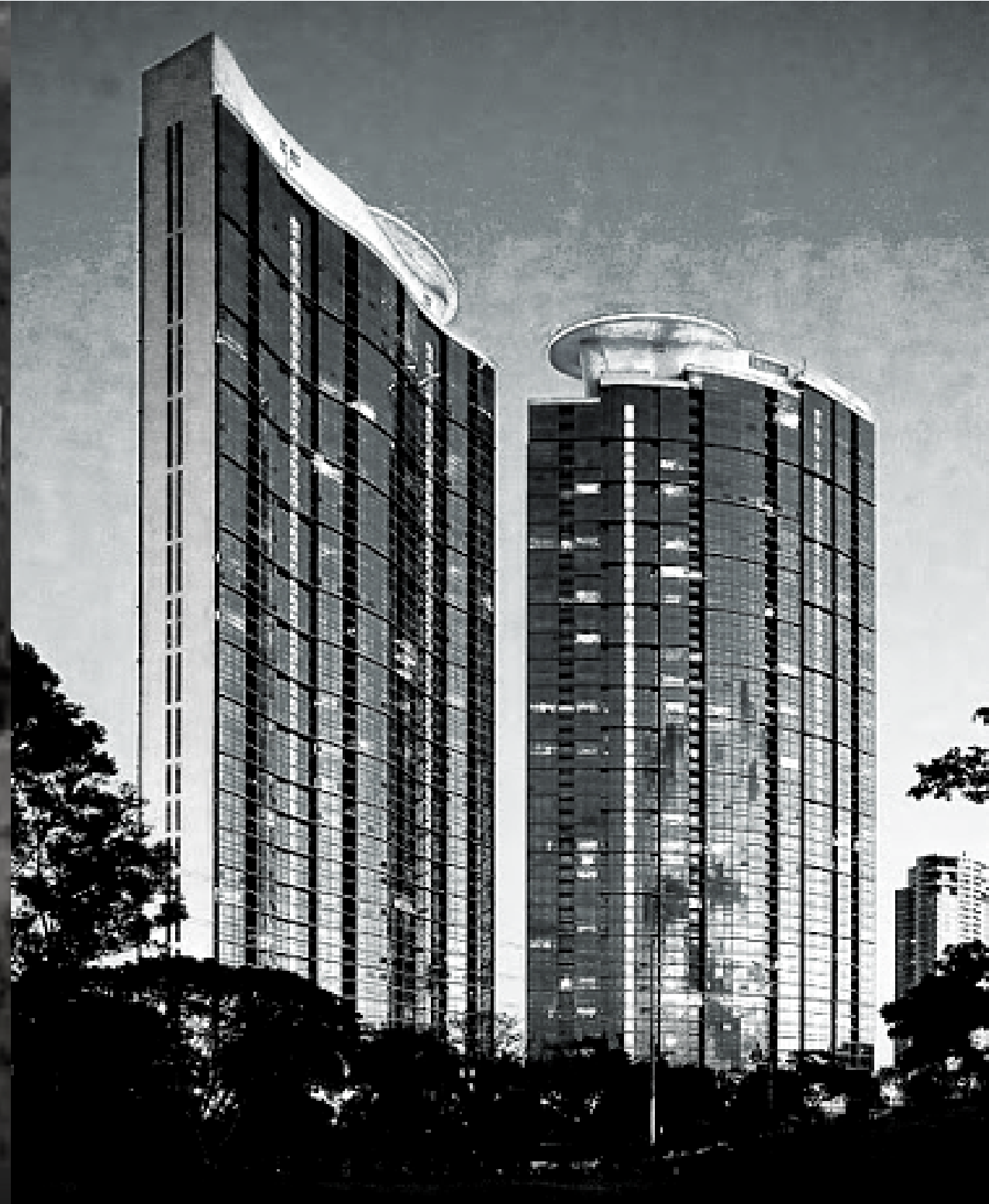
Pacific Plaza Towers
